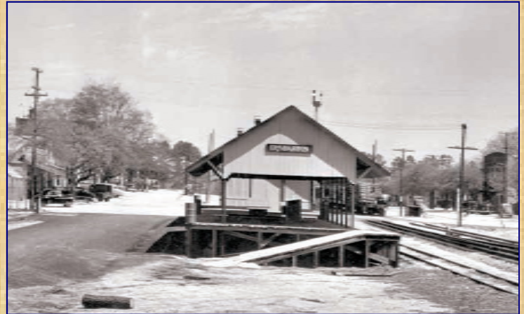
Dunbarton Grammar School above Left is the Dunbarton Train Depot Below, aerial photo of Dunbarton.
